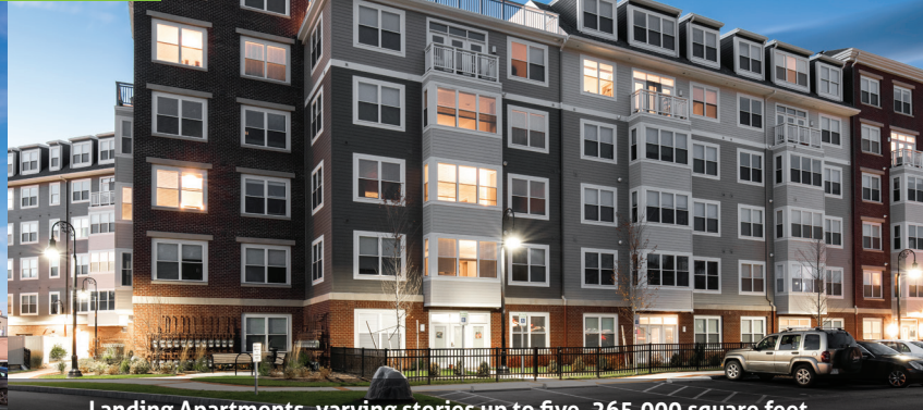
Landing Apartments, varying stories up to five, 265,000 square feet. Courtesy: Russell Scott Steedle & Capoine Architects, Inc.
