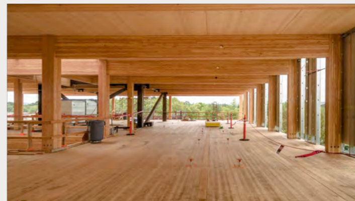
Above and below: First Tech Credit Union Headquarters under construction. With 5 stories of glulam and CLT, it's the largest mass timber building in the U.S. with 156,000 square feet of space. Seven workers erected the mass timber in 12 weeks.
