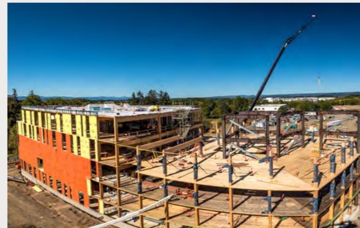
Above and below: First Tech Credit Union Headquarters under construction. With 5 stories of glulam and CLT, it's the largest mass timber building in the U.S. with 156,000 square feet of space. Seven workers erected the mass timber in 12 weeks.
